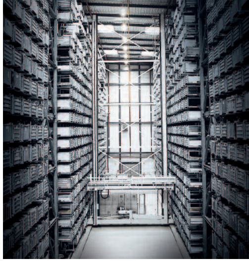
UNICOMPACT in an aluminum extrusion facility.
