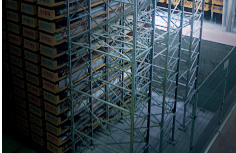
Honeycomb storage system in a pit.
