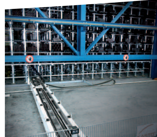
Buffer station at longitudinal side with 14 buffer locations.
