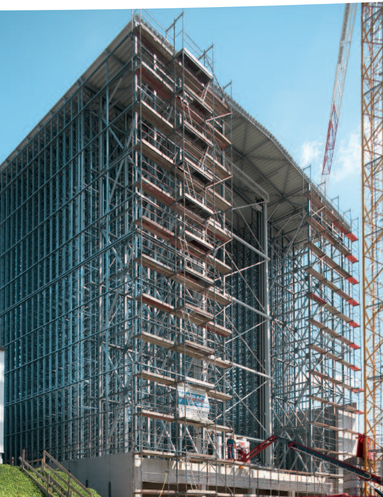
UNICOMPACT rack supported building during installation.
