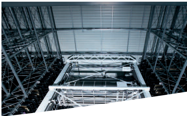
Roof connection of Honeycomb shelf block.
