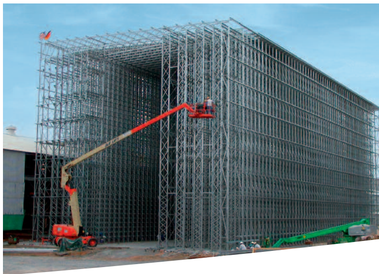
Completion of a Honeycomb steel structure with roof and wall connection.
